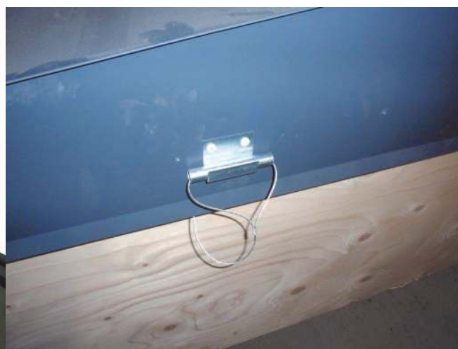
Manual opening (emergency opening)
